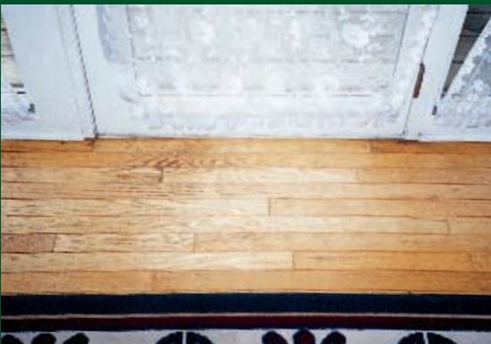
Dirty floors with finish totally worn off.
