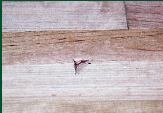
Dents (these usually require board replacement).
